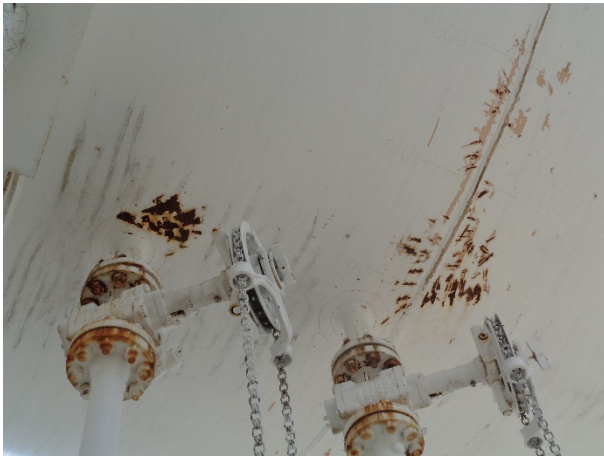
BOTTOM SHELL COATING DAMAGE, MINOR RUSTING
