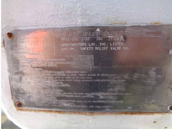
North PSV manifold Dataplate
