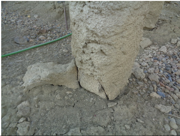
Minor fireproofing damage at base of supports
