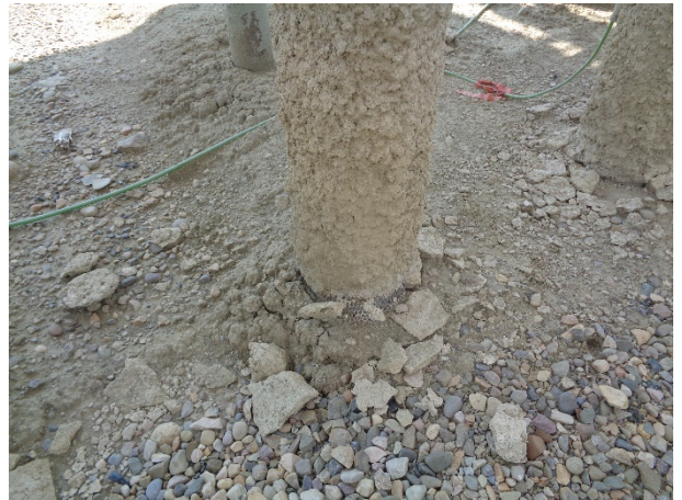
MINOR FIREPROOFING DAMAGE AT BASE OF SUPPORTS
