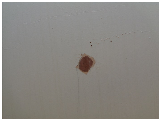
Shell paint deterioration to bare steel
