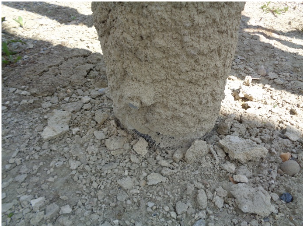
MINOR FIREPROOFING DAMAGE AT BASE OF SUPPORTS
