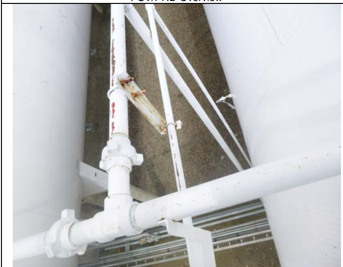
Small bore piping – Hammer unions & U-Bolts missing.
